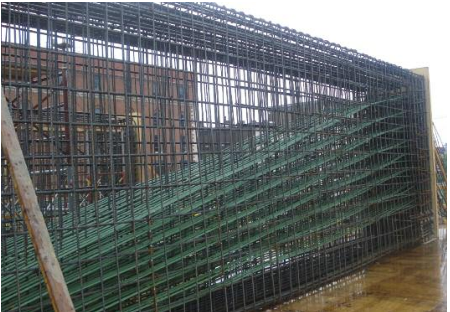
While the arena didn't need post-tensioning for its floor structure, it was necessary to have a column-free area to accommodate a practice court.
