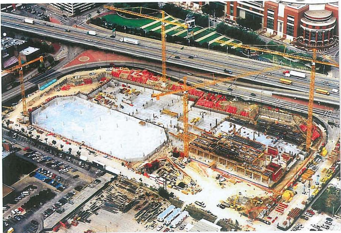
Fig. 2 – Construction of the moat for Lumiere Place Casino
